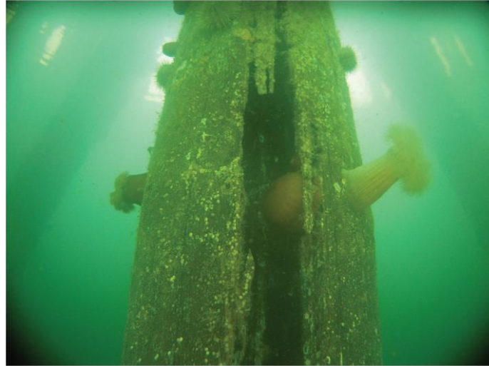
Fig. B-20. Underwater photograph showing hollowing of the interior of a timber pile from Teredo Source: Courtesy of Marine Solutions, Inc., reproduced with permission.
